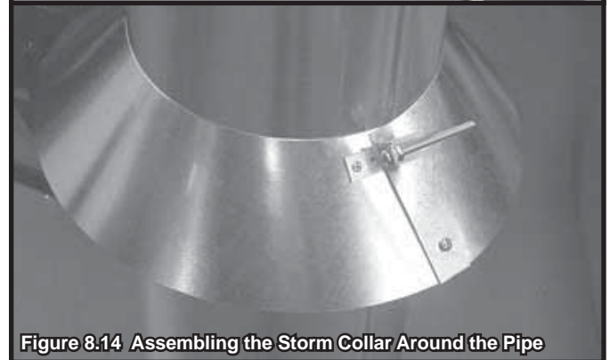
Figure 8.13 Assembling the Storm Collar
